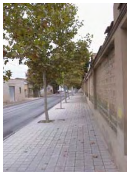
5. Vista general muro
